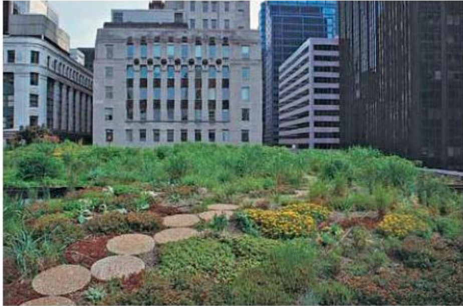
Intensive and extensive roof greening techniques can be combined on the same roof. Green roof atop Chicago City Hall.
