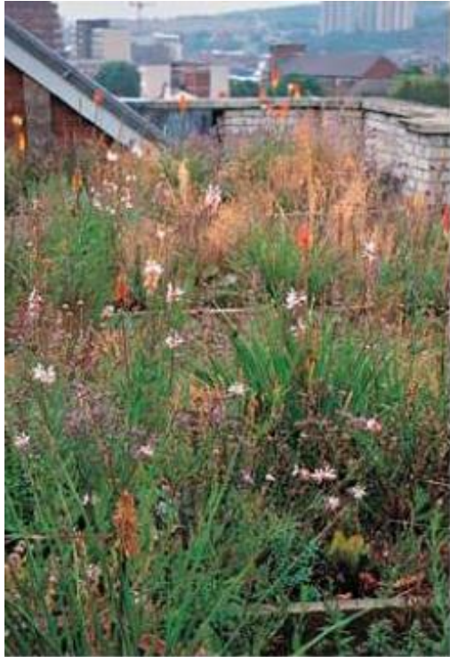
Semi-extensive roofs use the same lightweight technology and growing media as extensive roofs, but their slightly greater depth enables a wider range of plants to be grown. Planting design by Nigel
