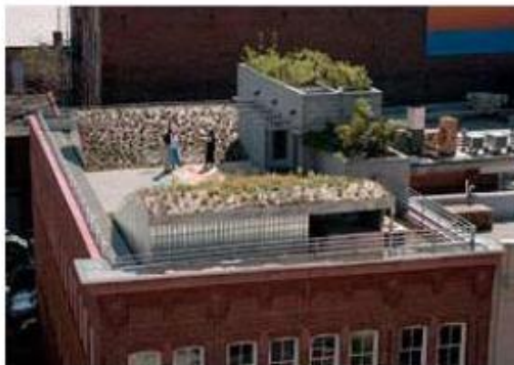
Intensive and extensive roof greening techniques can be combined on the same roof. Green roof atop Chicago City Hall.
