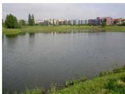
The restored water reservoir N1 – Stodůlky
